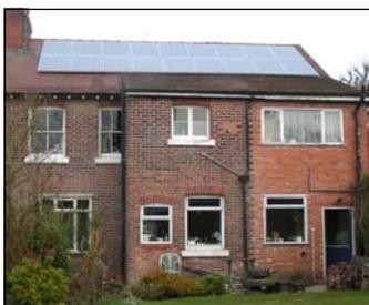
Another MESS member has installed an 18 panel system with a generating capacity of 3.9 kilowatts, the maximum for domestic installations. It is early days to see how much electricity is being fed back into the National Grid. On a dull rainy day the input was still 7.58 kwh which could return £3.41. On a hot sunny day the takings could reach
